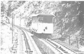
Penang Hill Railway.
